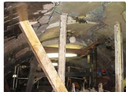
**Figure 5.** Image of the damaged section of Gibe II tunnel that failed in October 2006 under pressures that exceeded the design pressure by six times [6].
