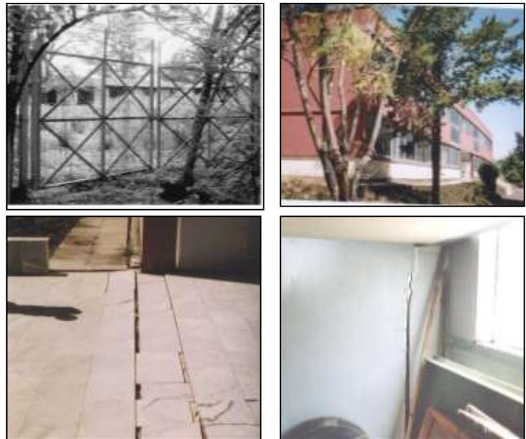
**Figure 7.** A closed and desolate rice-processing factory in the original **Tana-Beles** project [9]. The other three pictures show foundation Failure of three buildings at the **Akaki Spare Parts Factory** [10].
